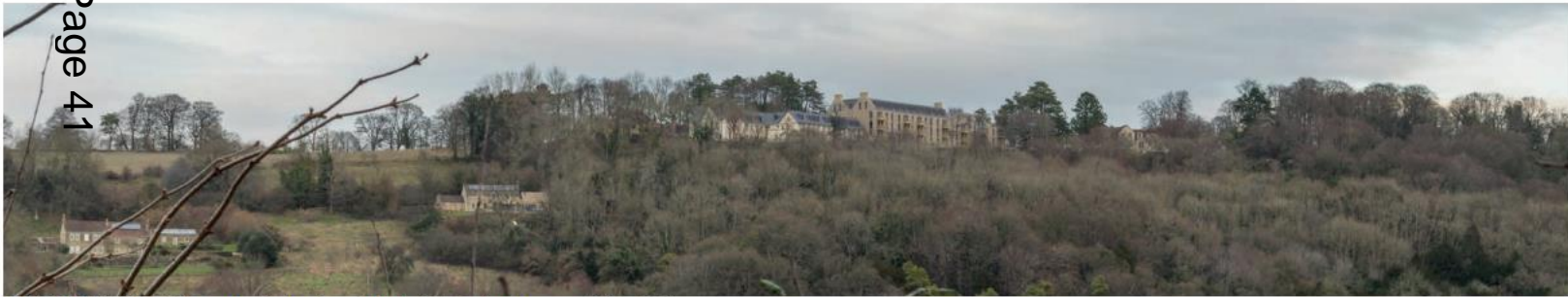
PROPOSED WINTER, ZOOMED IN: Photomontage View from Crowe Hill, Limpley Stoke - planting shown as year 15 (at scale@A3)
