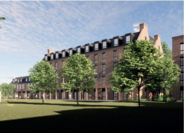
3. View showing the southern extension from north block A
